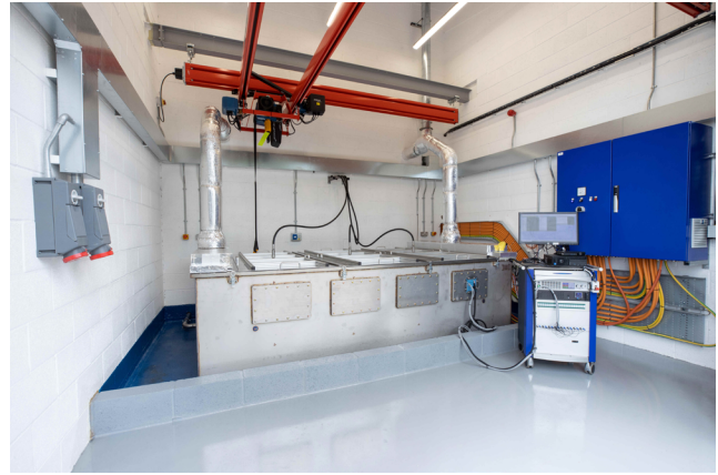
>> Battery pack test facility
